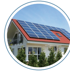
Private house/villa area
